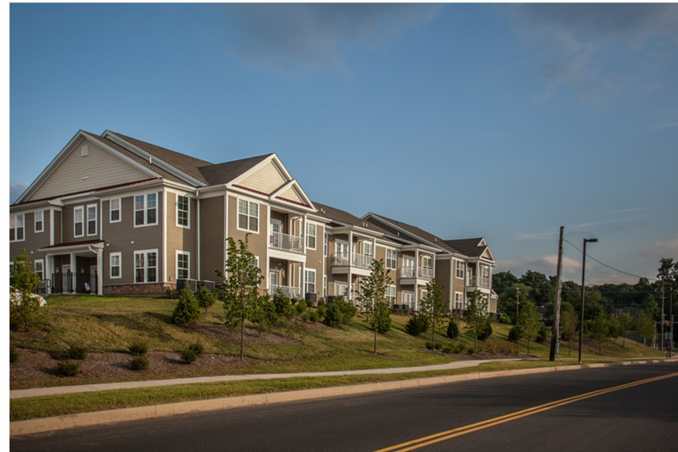
3 | FLATS REPRESENTATIVE PHOTO Scale: NTS
