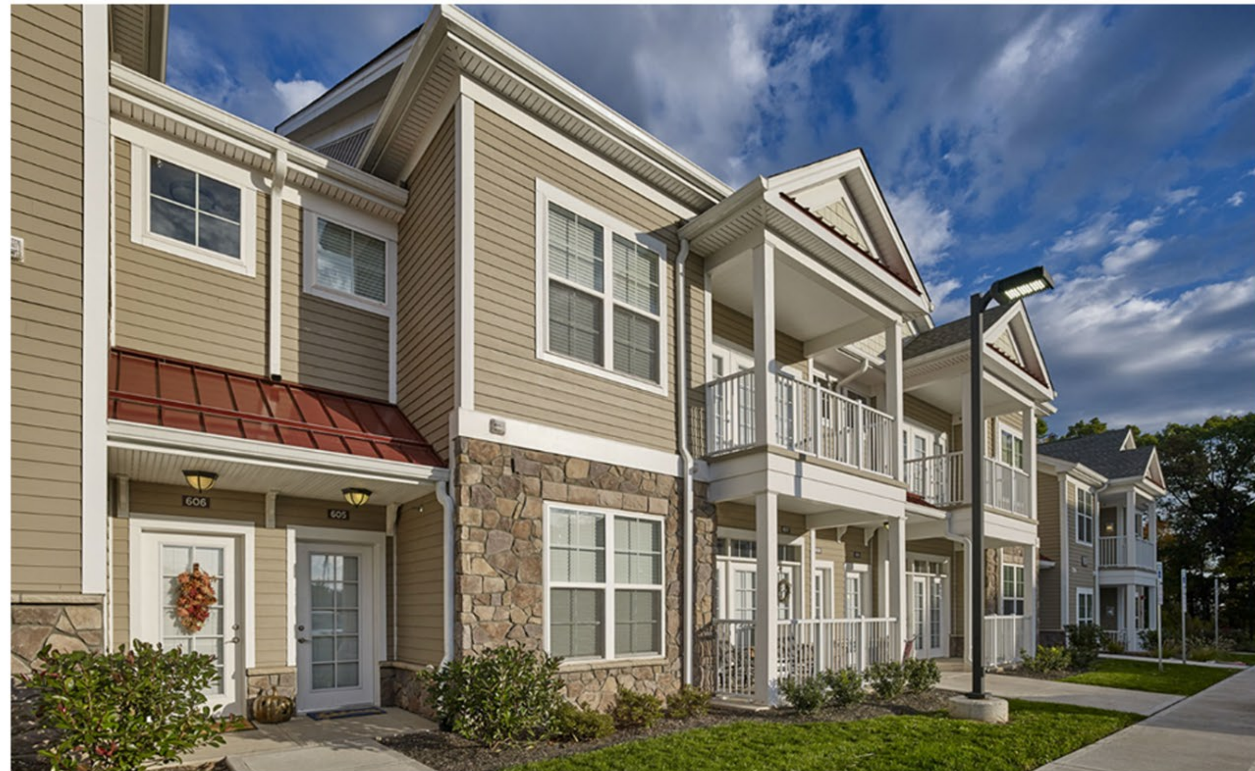
2 | FLATS REPRESENTATIVE PHOTO Scale: NTS
