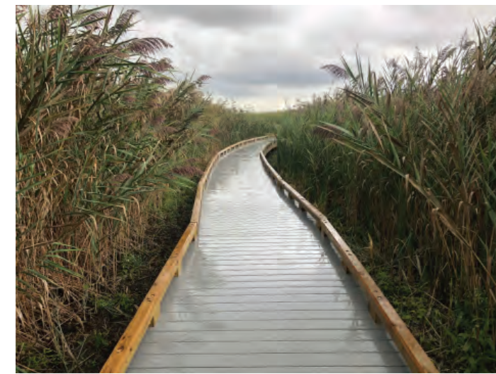
WETLAND BOARDWALK WITH CURBING
