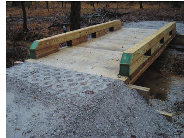
WOODEN PEDESTRIAN BRIDGE WITH CURBING
