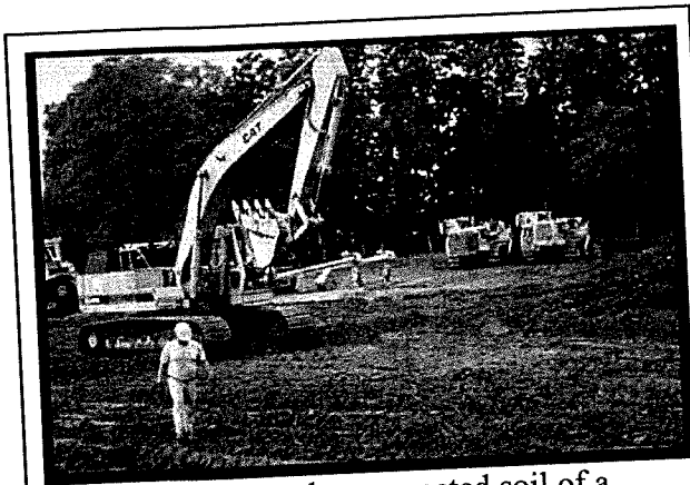
Fig. 14. The severely compacted soil of a temporary construction yard used daily by heavy equipment for four months; shown before deep ripping, topsoil replacement, and decompaction.
