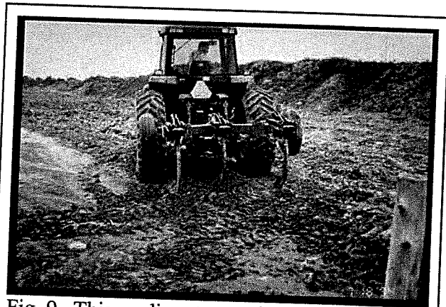
Fig. 9. This medium tractor is pulling a 3-shank deep ripper. The severely compacted construction access corridor is narrow, and the 120 hp tractor is more maneuverable for Phase 1 deep ripping (subsoil fracturing), here.
