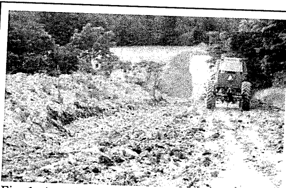
Fig. 1. A typical deep ripping phase of this practice, during the first in a series of progressively deeper “rips” through severely compressed subsoil.
