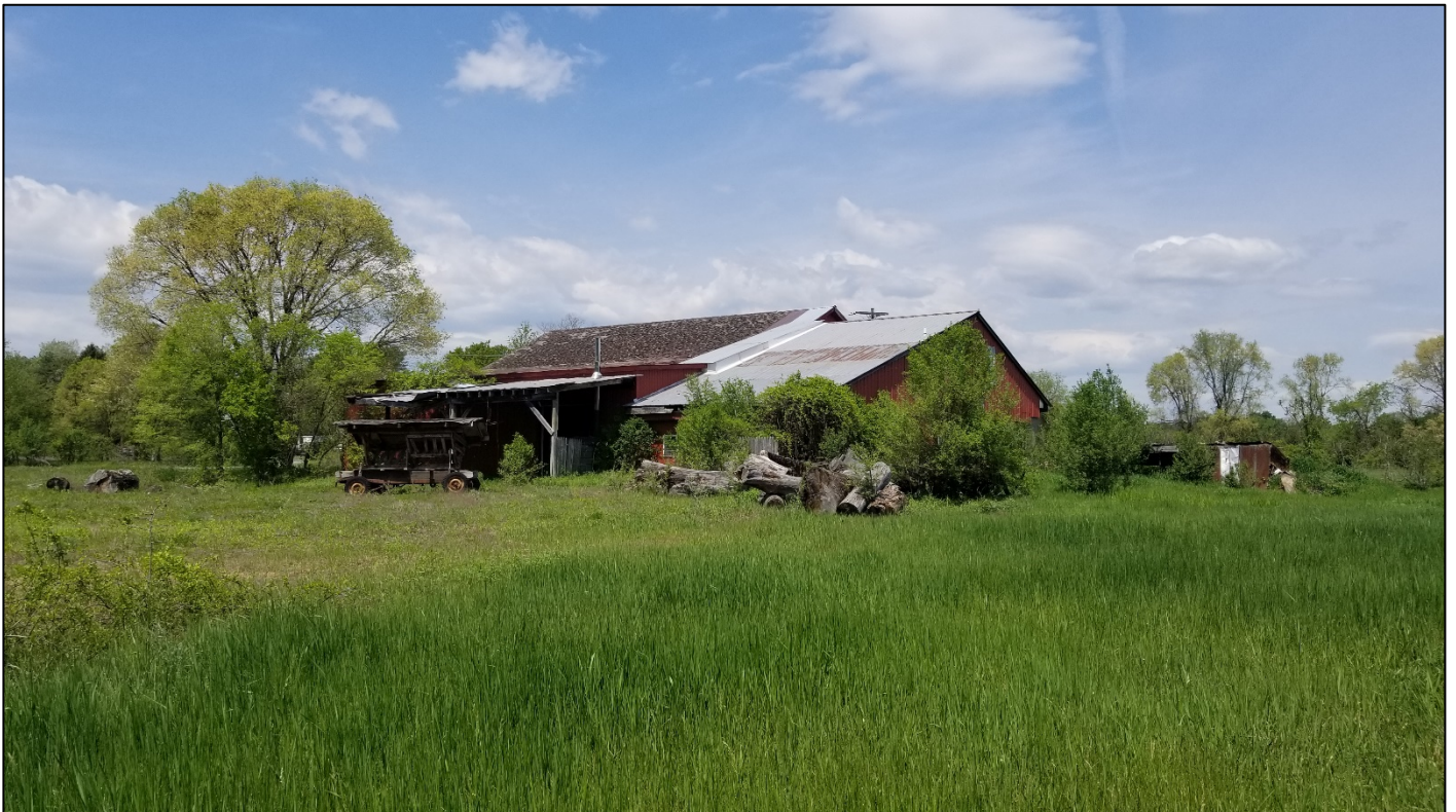
Photo 20. Looking northwest at existing conditions.
