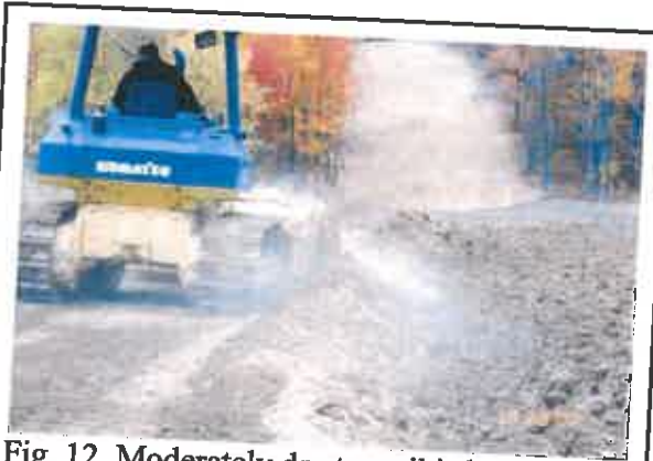
Fig. 12. Moderately dry topsoil is being replaced on the affected site now that Phase 1 deep ripping of the compressed subsoil is complete.
